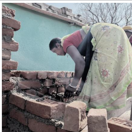
Mason training student at worksite
